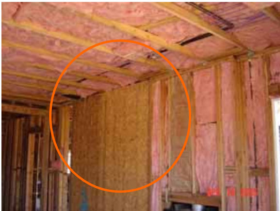
Figure 1. Exterior wall showing shear paneling on interior wall.
