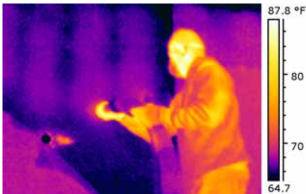
Figure 9. Thermal of contractor blowing in insulation, wall being insulated.
