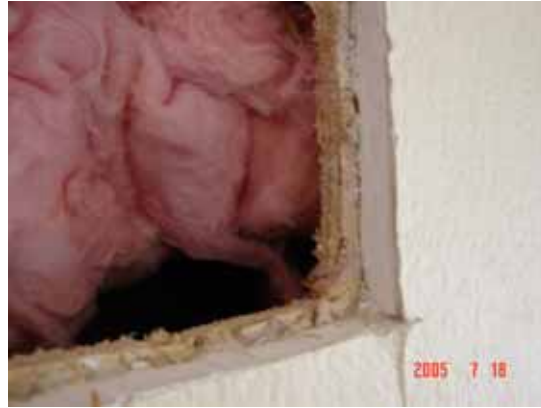
Figure 6. Close up of hole cut showing insulation threads on shear panel.
