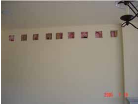
Figure 5. Nine holes cut in drywall/shear panel
